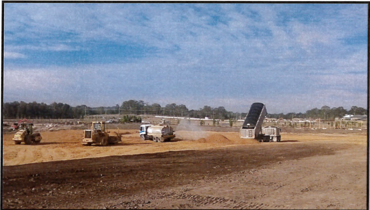
Picture 3: Site Earthworks Filling Operations
