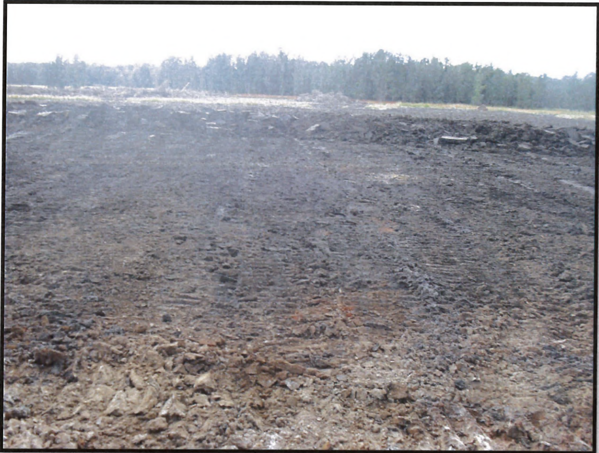
Picture 2: View of the Stripped Surface Prior to the Placement of Fill
