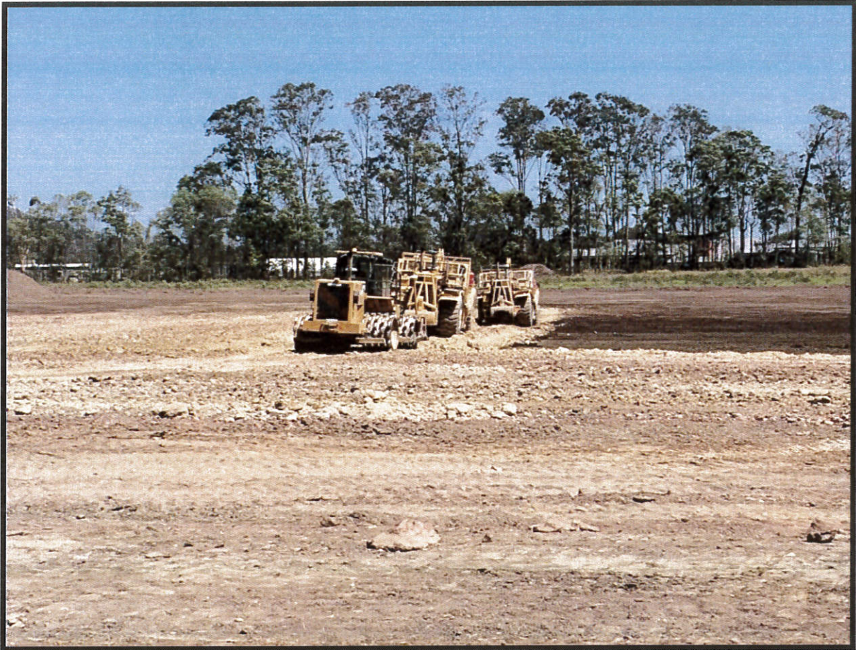
Picture 3: Site Earthworks Filling Operations
