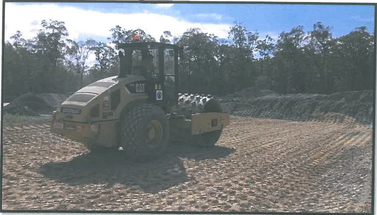
Picture 3: Site Earthworks Filling Operations
