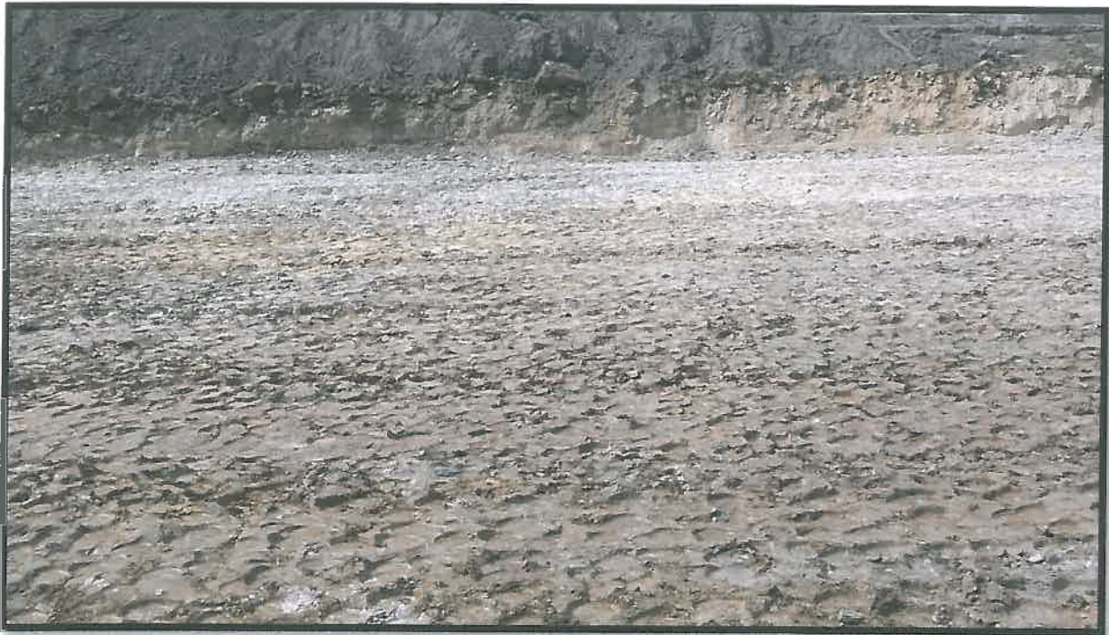
Picture 2: View of the Stripped Surface Prior to the Placement of Fill
