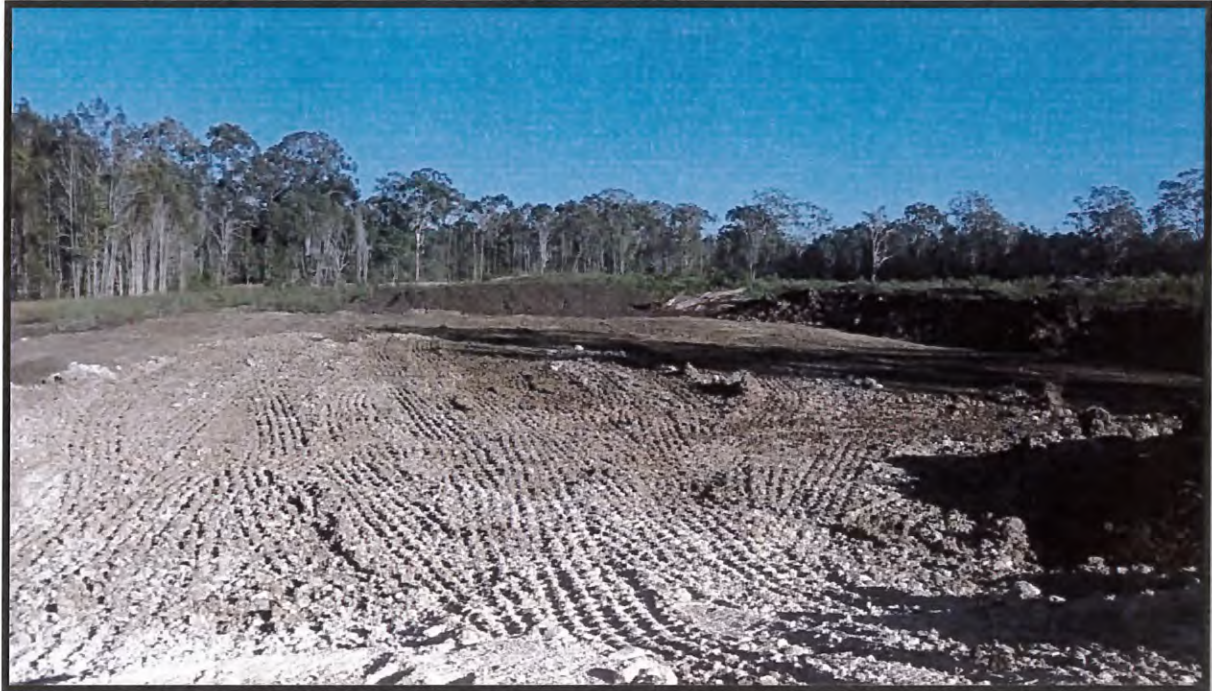
Picture 2: View of the Stripped Surface Prior to the Placement of Fill
