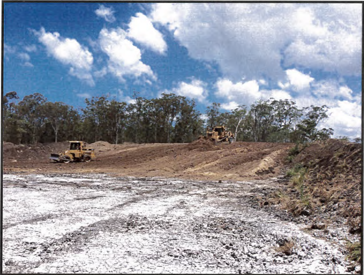
Picture 3: Site Earthworks Filling Operations
