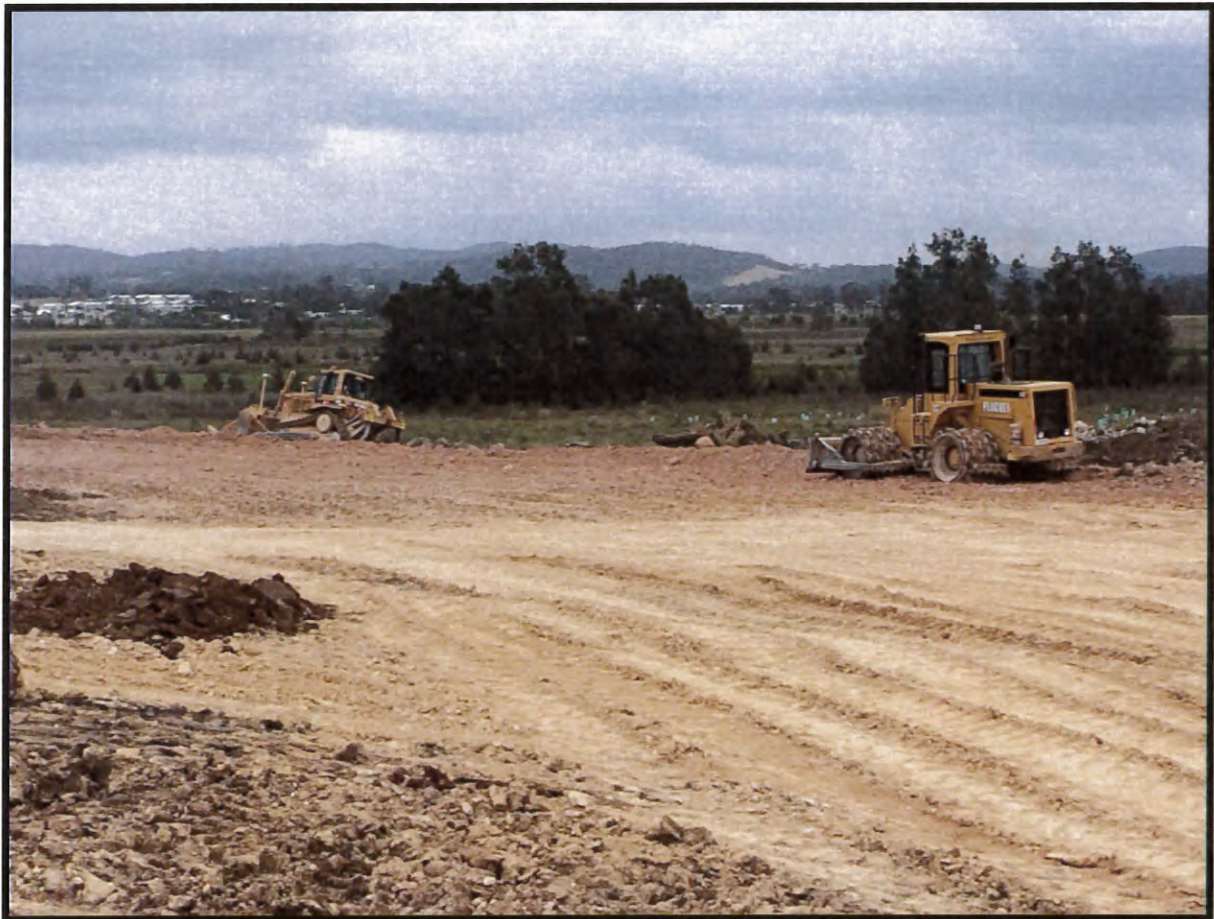
Picture 3: Site Earthworks Filling Operations
