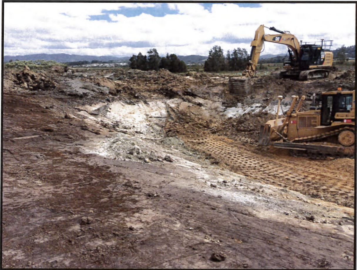
Picture 2: View of the Stripping Operations Prior to the Placement of Fill
