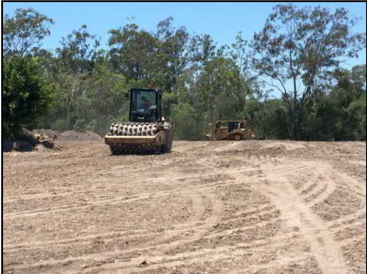
Picture 3: Site Earthworks Filling Operations
