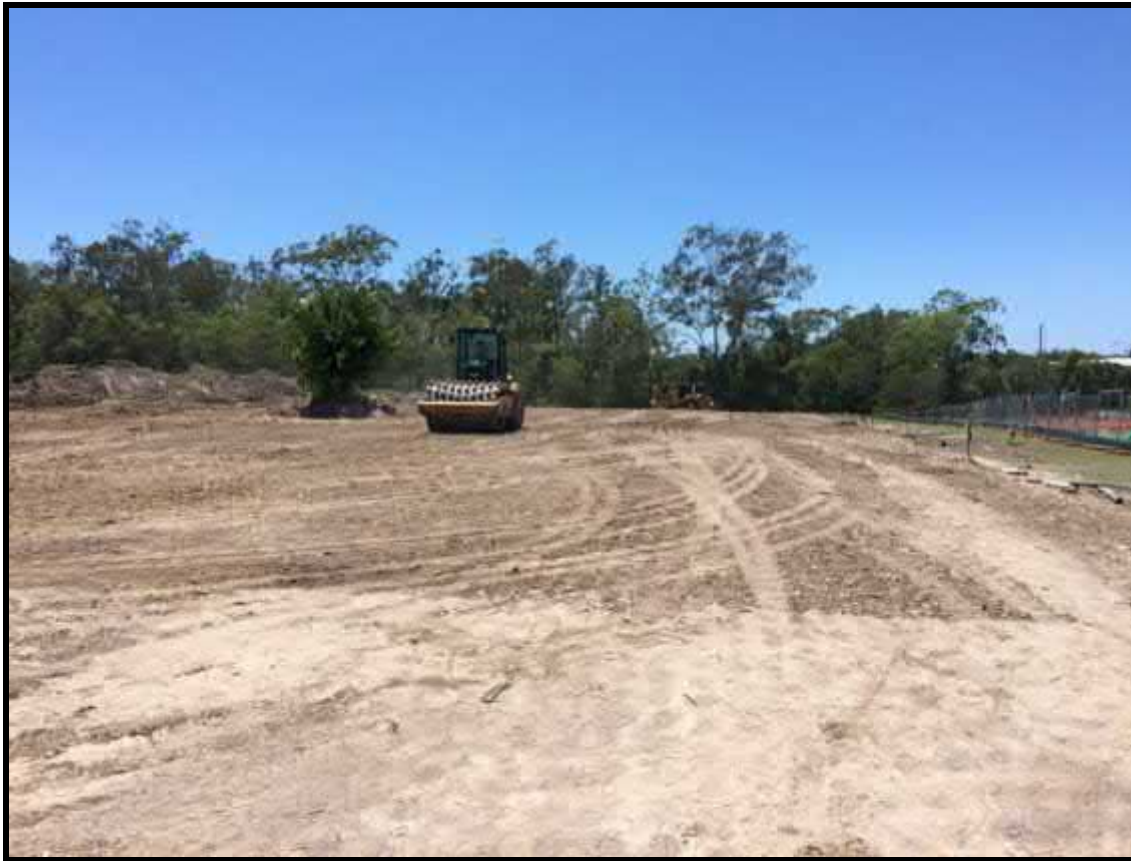
Picture 2: View of the Stripped Surface Prior to the Placement of Fill
