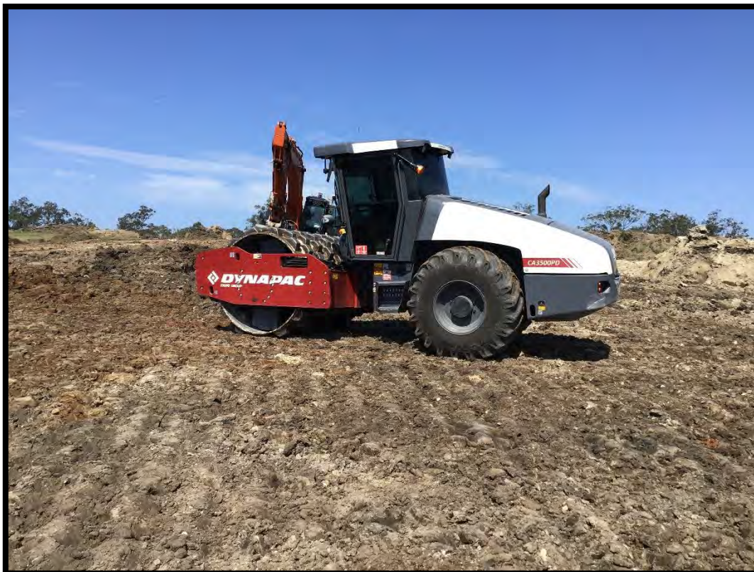
Picture 8: View of the Site During Construction
