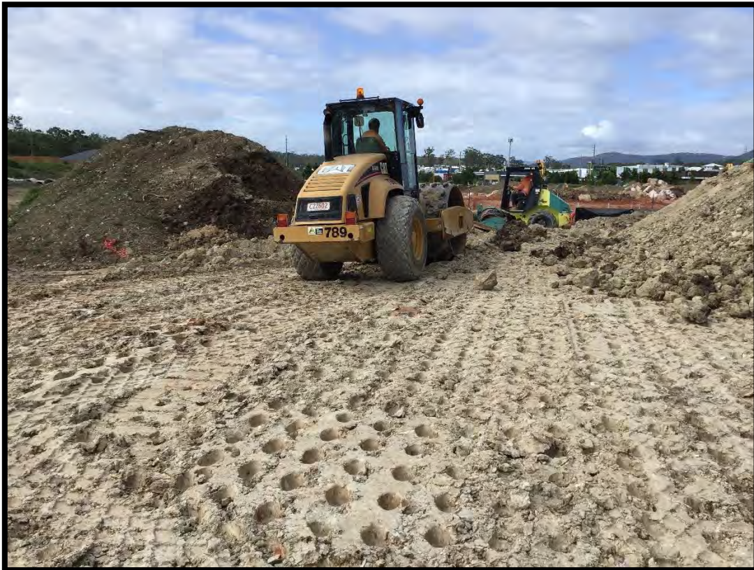
Picture 7: View of the Site During Construction
