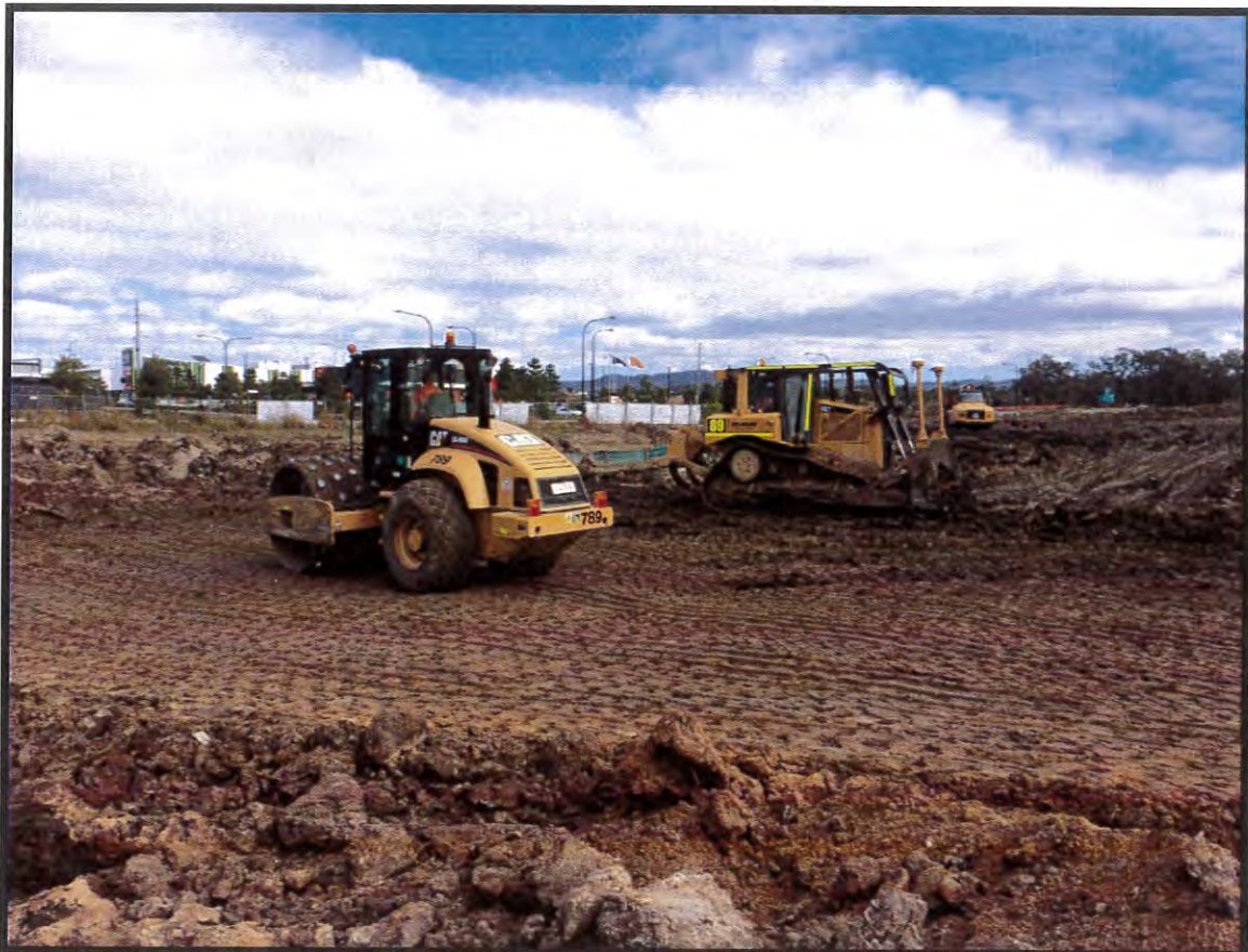
Picture 3: Site Earthworks Filling Operations
