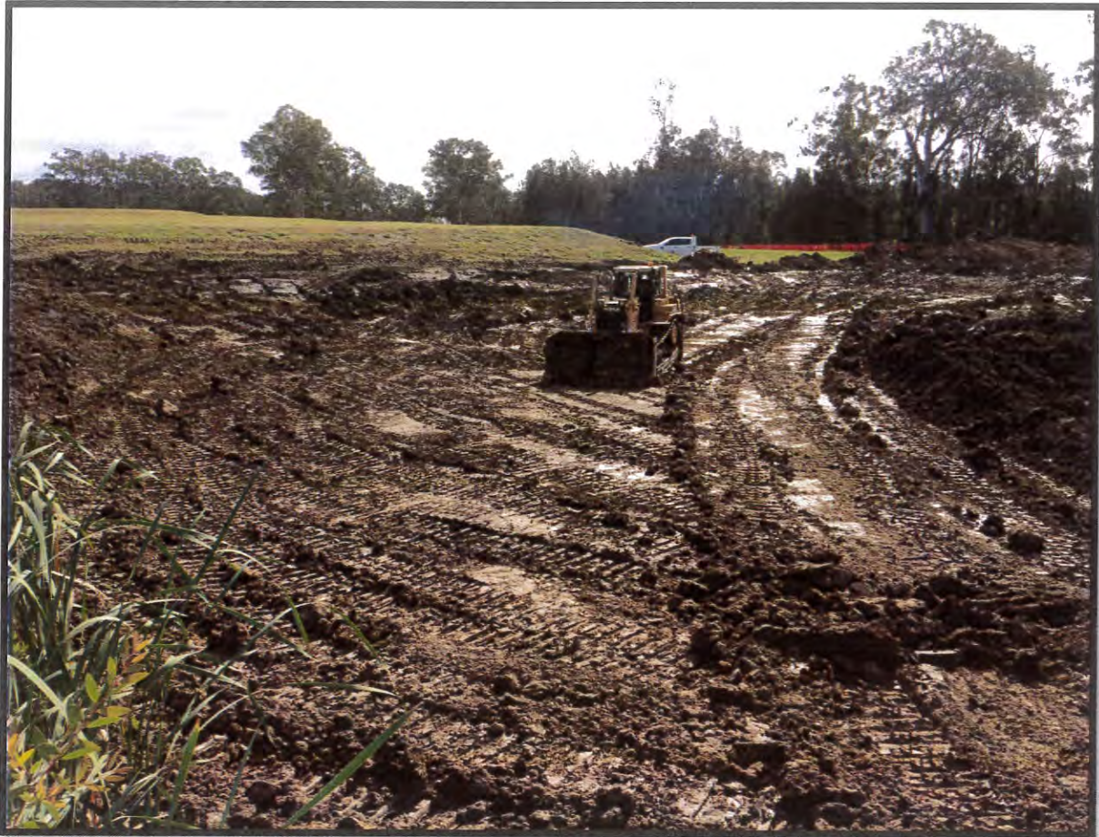
Picture 2: View of the Stripped Surface Prior to the Placement of Fill
