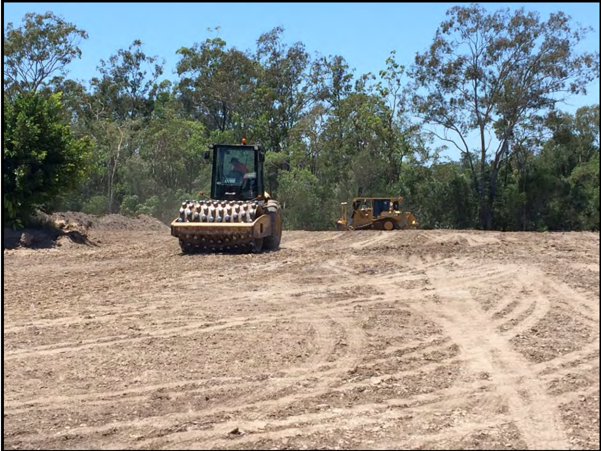
Picture 3: Site Earthworks Filling Operations
